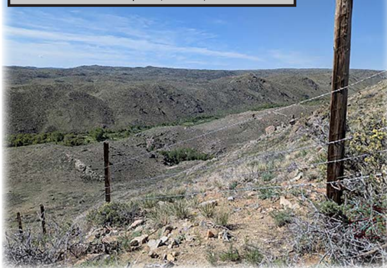
New wires on re-used posts, Thorne/Williams WHMA.
