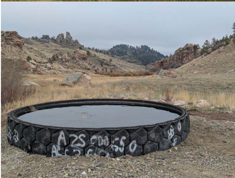
Image 3: Hay Canyon, After Installation. October 2025.
